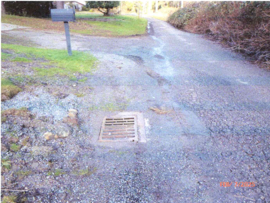
EXISTING CATCH BASIN ON 97TH AVENUE S.E.
